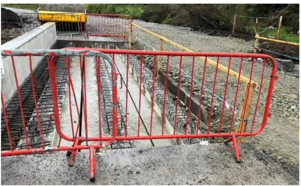
Figure 25 Photo of precast MY1 deck beams and edge beam, prior to in-situ concrete slab pour
