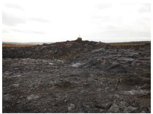
Figure 118 T16 photo showing incomplete turbine excavation works on solid bedrock
