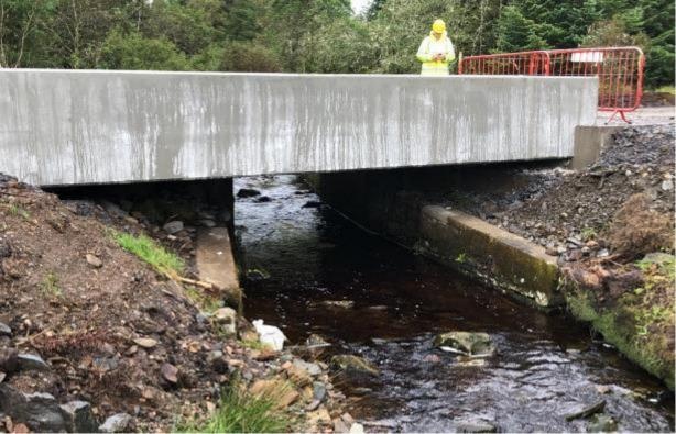
Figure 24 Photo of precast edge beam spanning beyond the original wing walls and original bridge
